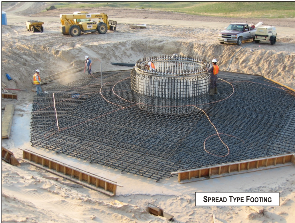
Figure 2-6 Turbine Foundations
