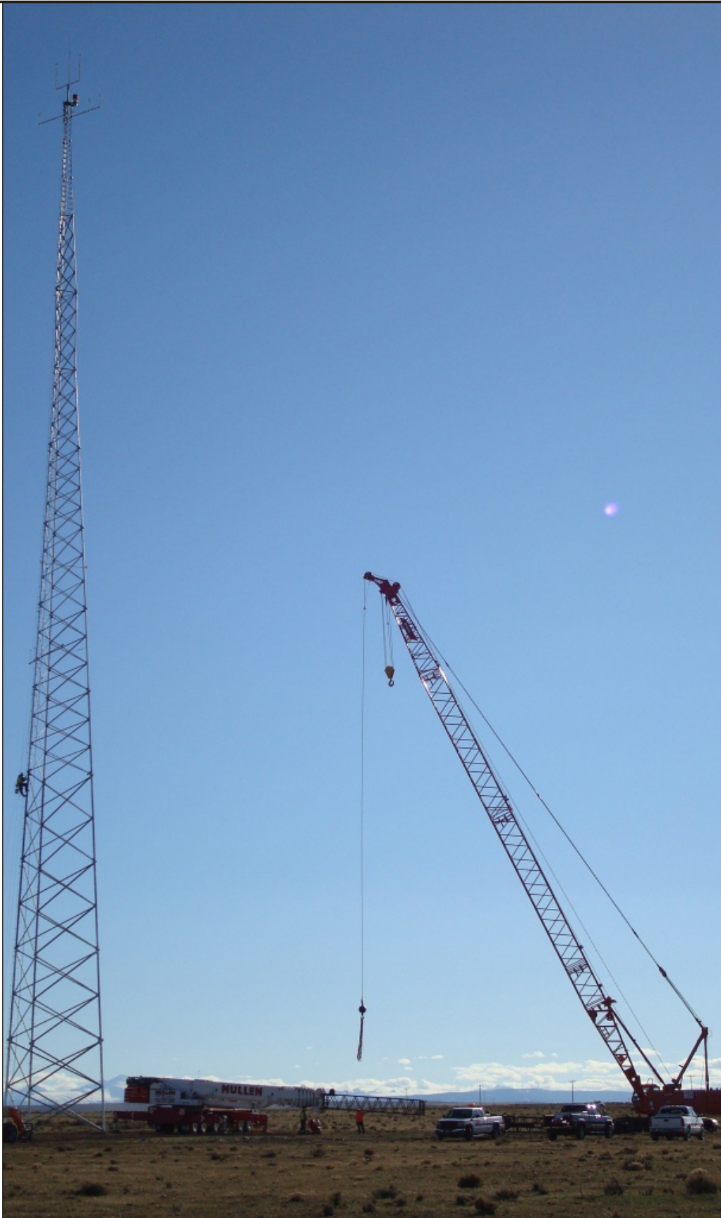
Figure 1-15 Typical Meteorological Tower
