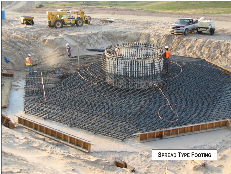
Figure 1-13 Typical Turbine Foundations
